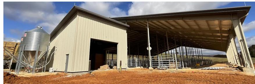
Description: 20 stall cattle housing facility to conduct feed studies. Includes cattle working area, loading chutes, feed mixing room, lab space, 4 grain bins, and 4 covered bulk commodity storage bins.
